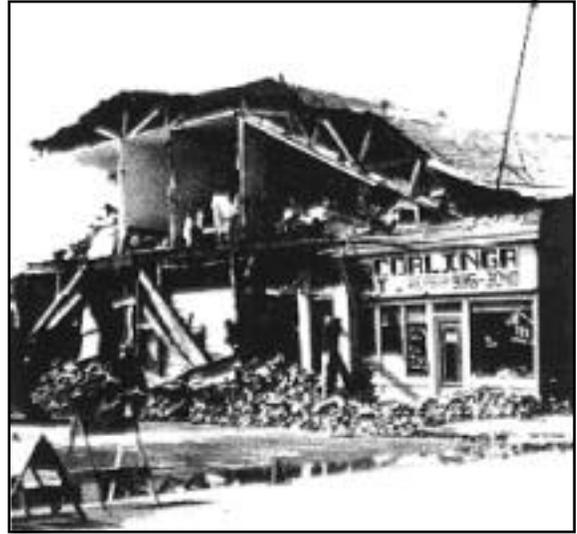
Photo 2. Masonry structures with little or no reinforcement, such as those in the Coalinga business district, usually sustain the greatest damage during an earthquake. Photo by James Stratta.
