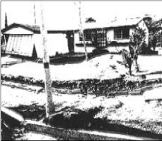
Photo 1. Single story wood frame houses usually stand up well to earthquake shaking. Even though fault rupture extends beneath this structure, it did not collapse during the 1971 San Fernando earthquake. The garage, however, with the large opening in the front, did yield to the horizontal shaking. Photo by R. Castle, courtesy of U.S. Geological Survey.
